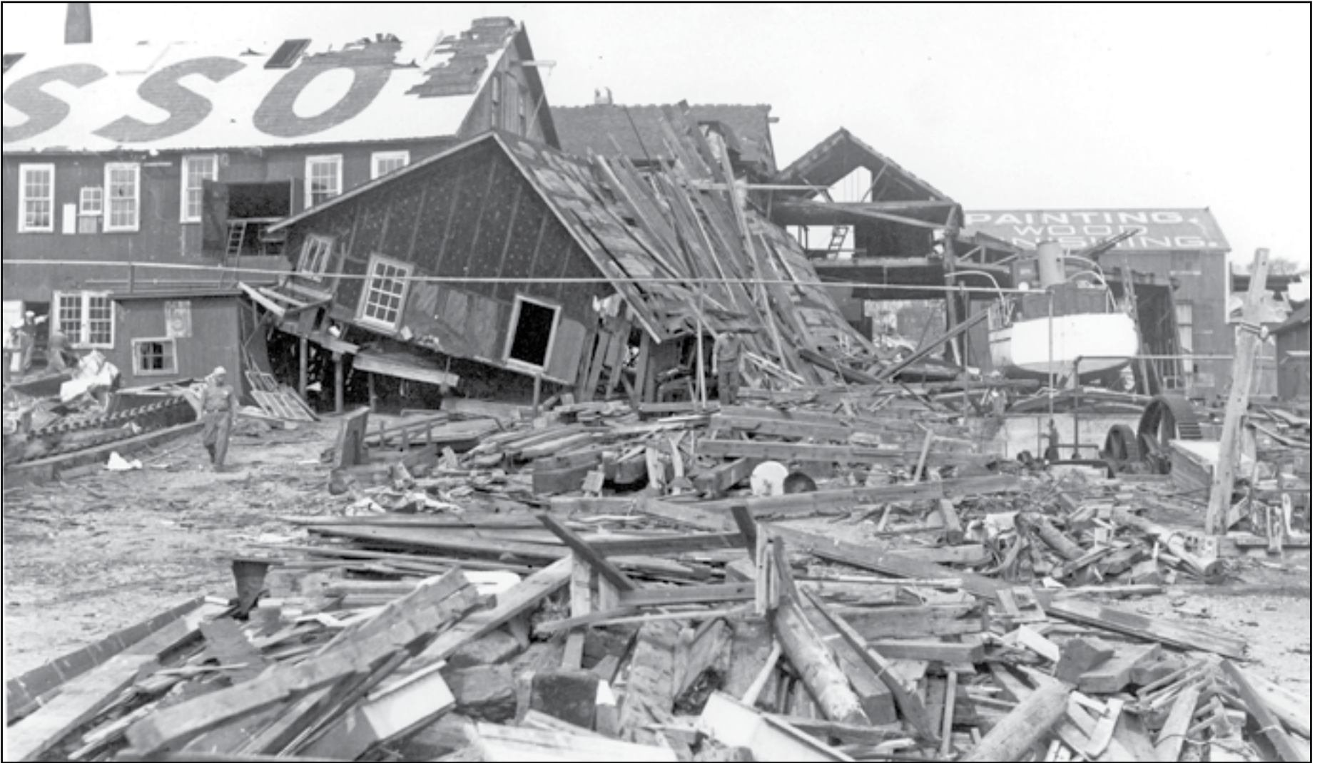
Greenport Basin and Construction Company, Railways #2 and #3. Photo from the PBS archives, courtesy of Mike Richter.
