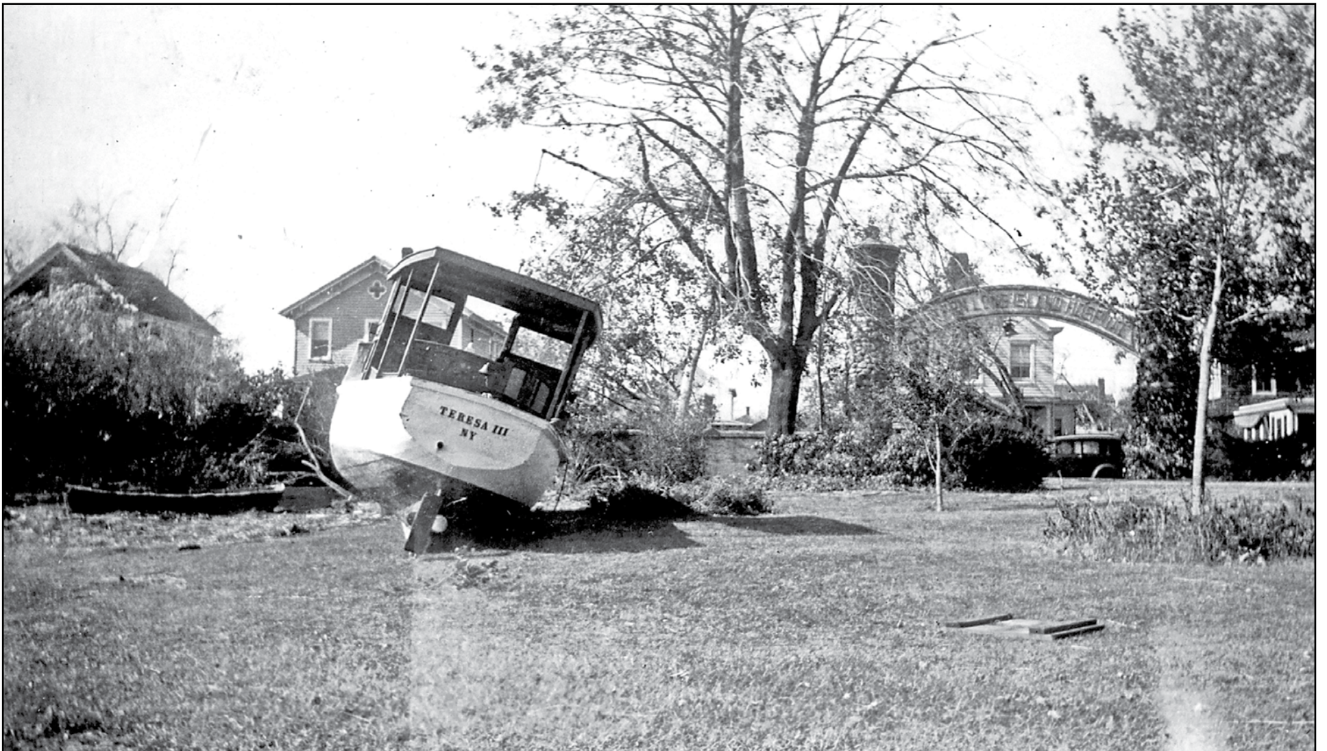
In the aftermath of the big blow of 1938, the "Teresa III" sits high and dry at the gate of the Eastern Long Island Hospital in Greenport. As Puerto Rico and Florida dig out of the carnage delivered by Ian, we are reminded of the misery these storms create.
