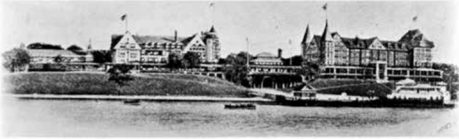
Manhasset House, Shelter Island
