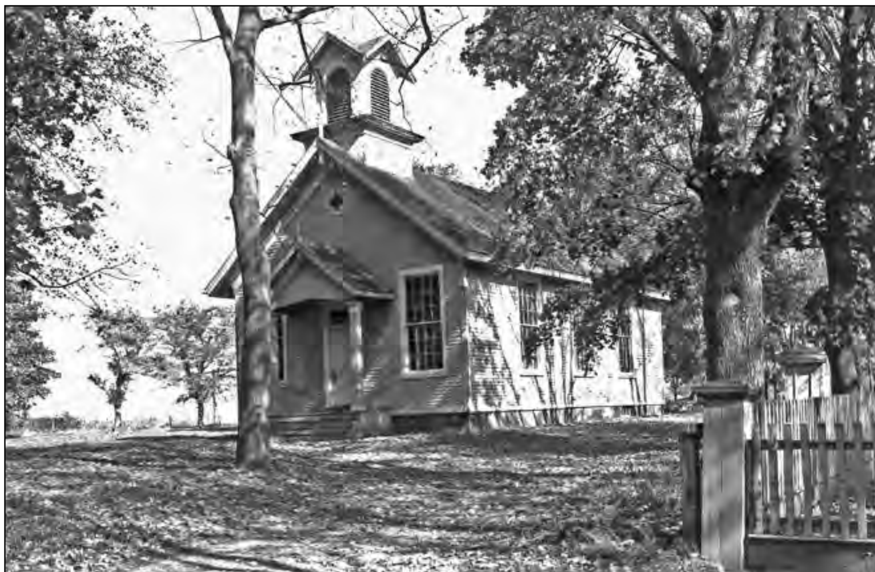
The Academy building with outhouse, circa 1900. The cupola ledge was accessible through a screen-hinged door in the back. Built in 1867, the building served as a preparatory study for college and higher learning, and later a school for commercial training. (photo from the Peconic Bay Shopper archives.)
