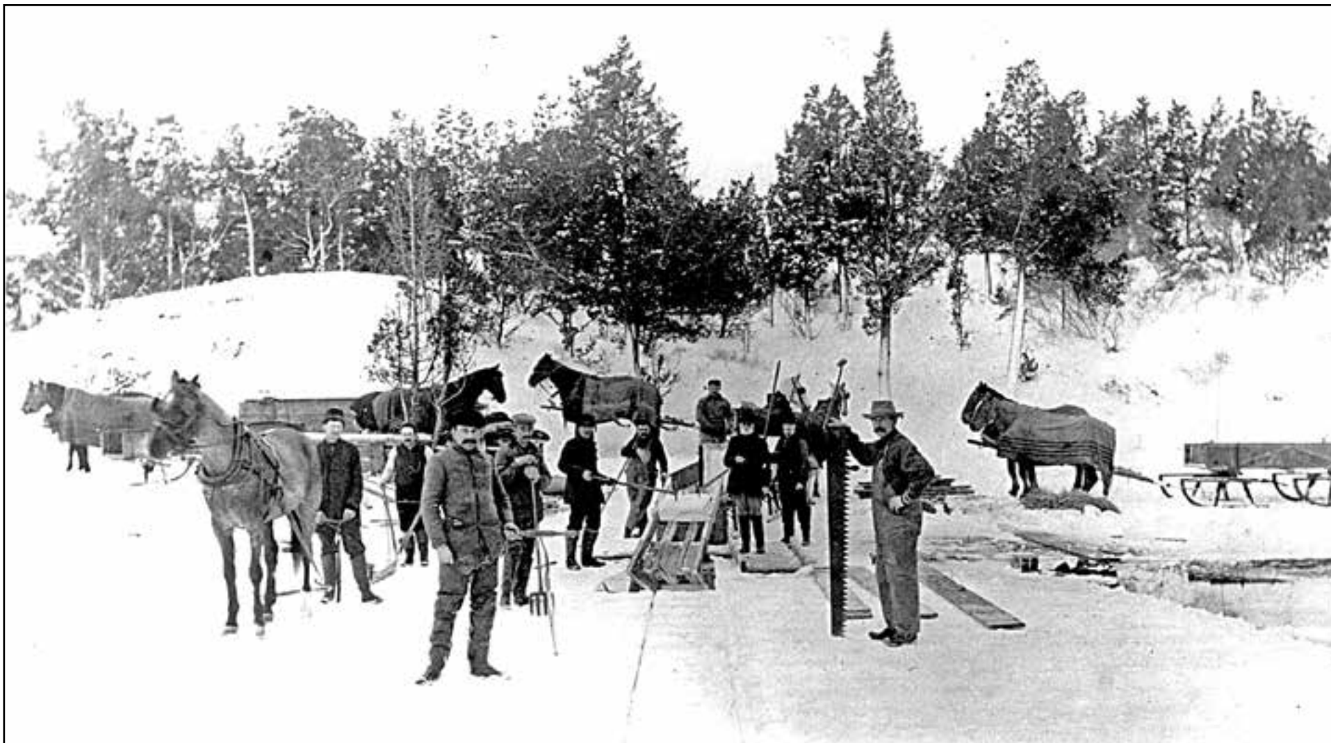
Ice cutting days on East Marion Lake shows a horse-drawn snow scraper on the left. An ice cake is being pushed up the wooden ramp to be loaded onto the horse-drawn sleds. The ice saws were quite heavy and long (almost as tall as the man on the right).
