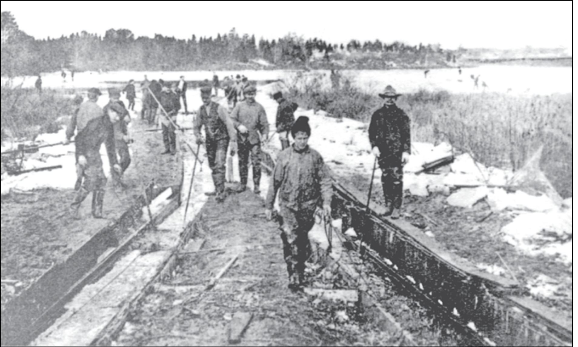
This ramp leads up to the ice house located between East Marion Lake and the Bay. Note the long line with grapple on the left being used to haul the ice cakes.
