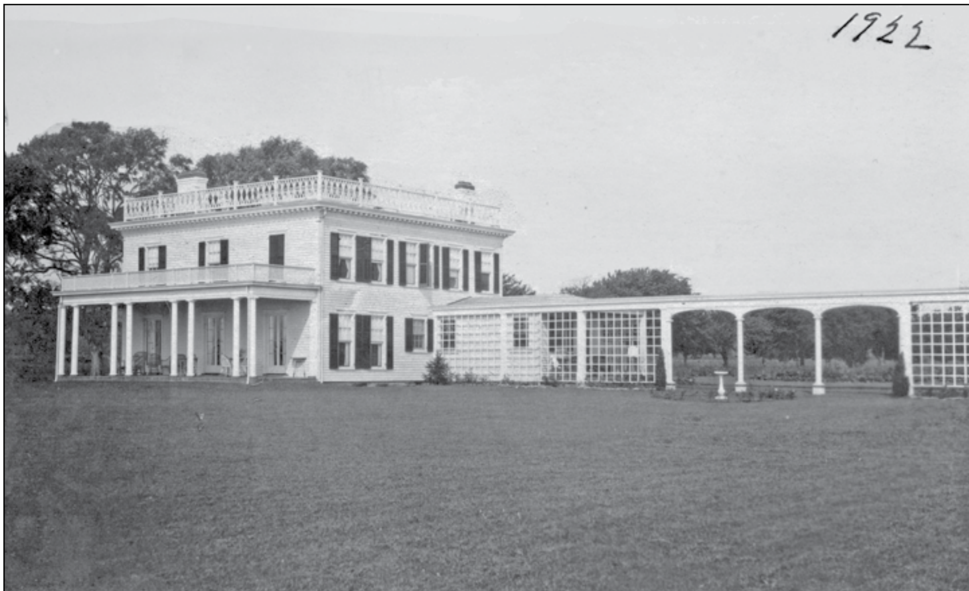
And now it's mid-summer 1922. The columns of the new front porch are in position. As a result of World War II, the front porch was enclosed to make a three seasons Florida Room, as gas ration coupons did not allow enough gasoline to go to Florida in winters. Note the single story bump out behind the rose trellis. This was the new kitchen as this hotel building had no kitchen when it was up on the Main Road. Also note the shorter windows – they are the windows from the hotel's third floor. The building was ultimately sheathed in three-quarter inch bottoms of clapboard. Still on the building today. But Mr. Lang found painting the house every two years to be too much maintenance, and second sheathed the house in eight and one-half inch reveal white cedar shingles. Our son Ryan just redid the second floor shingles of the side facing the bay summer before last. Found these twenty-four inch long shingles in the mid-west.
