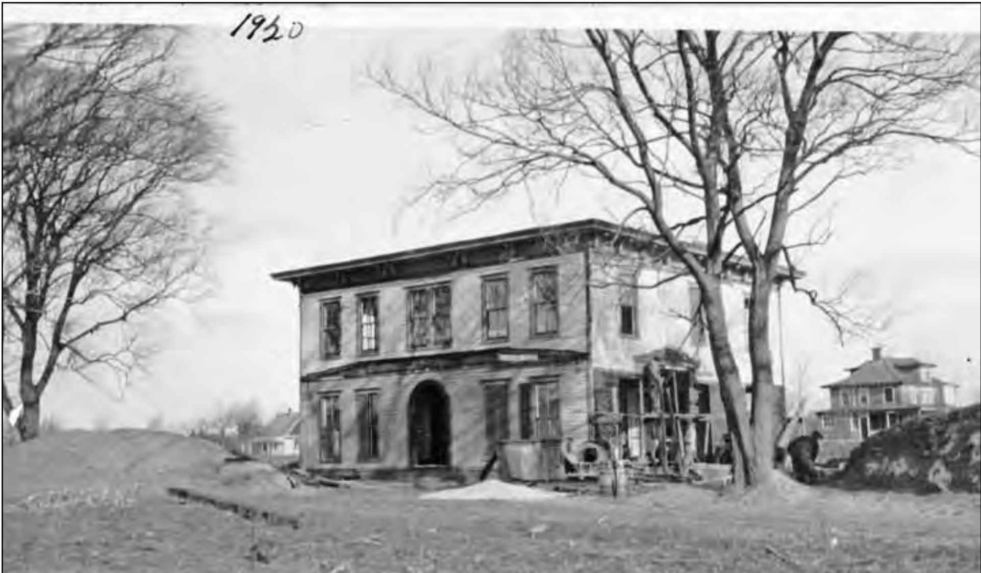
Looking from the south to the north, is the front façade minus the full width covered porch. The last vestiges of Victorian architecture are the semi-circular top of the main entrance, the pairs of brackets under the eaves of the roof edges (the roof was all yankee guttered, and still is), and the window sashes are still two-over-two lights. In the foreground is a big, steel-strapped wooden barrel just behind a manual water well pump. It was the only source of water for men and horses then. The pump seems to have gone sometime after 1925. Note the large mounds of dirt. These are the spoils from digging the cellar before the building was positioned. Later, this dirt was spread out around the bay front and sides of the house. This gave the house an extra one & one-half feet of elevation which 82 years later prevented inundation of the cellar and its mechanicals from Superstorm Sandy. More than two acres of the front lawn were under bay water during Sandy's high tide.
