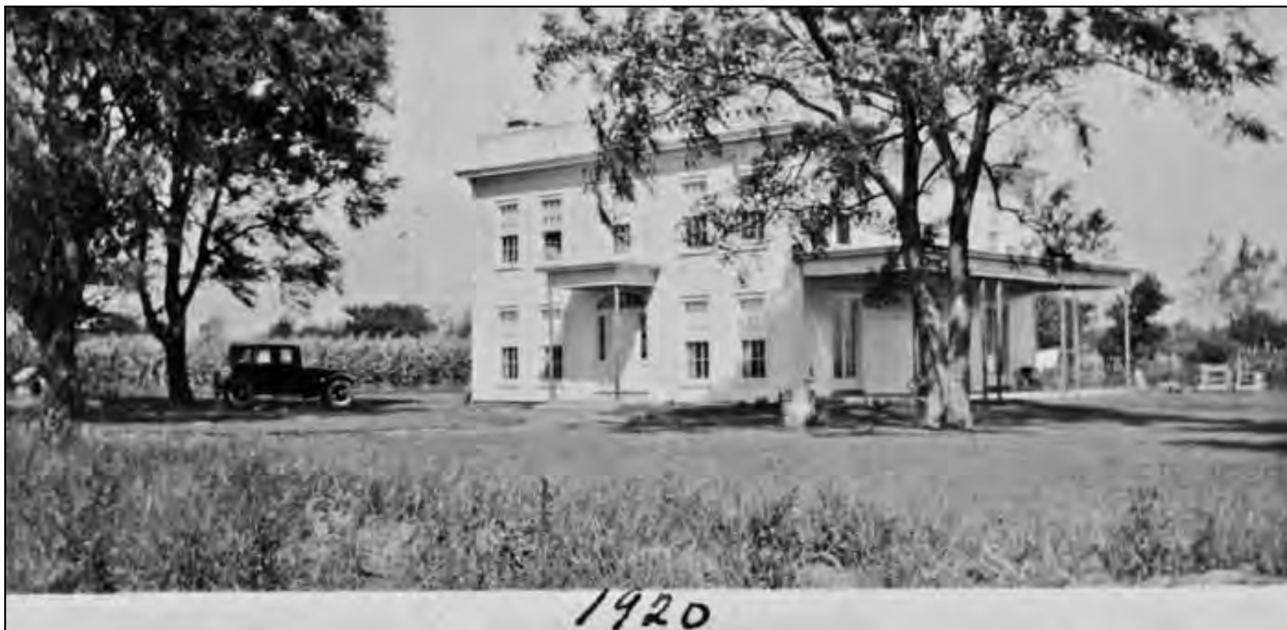
The hotel in its new dress. By late July – early August 1920, the architectural conversion from Victorian to America’s first architectural style – Federal – had been completed: the elliptical fan light over the front door, the leaded glass side lights, all the sashes of the windows had their mortise and tenons reopened so that six lights per sash could be mounted. They saved and reused everything they could one hundred years ago. Note the height of the corn stalks to the left of the house, Robert Lang’s 1919 Lincoln, and just at the edge of the photo the guard dog’s dog house, which still exists today.
