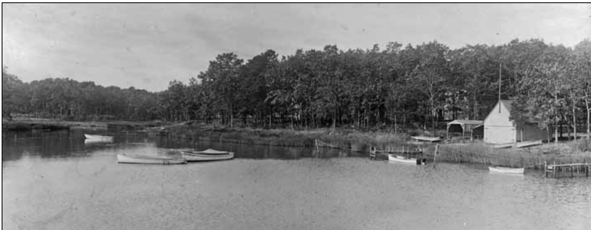
The Cove west of the Westphalia Avenue Bridge. This popular ice-skating area no longer exists, having been filled in with dredged sediment from the creek. (M-L Library)
