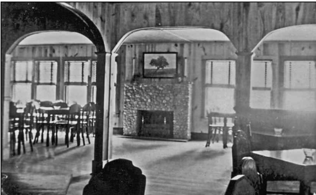
A better view of the fireplace room.
