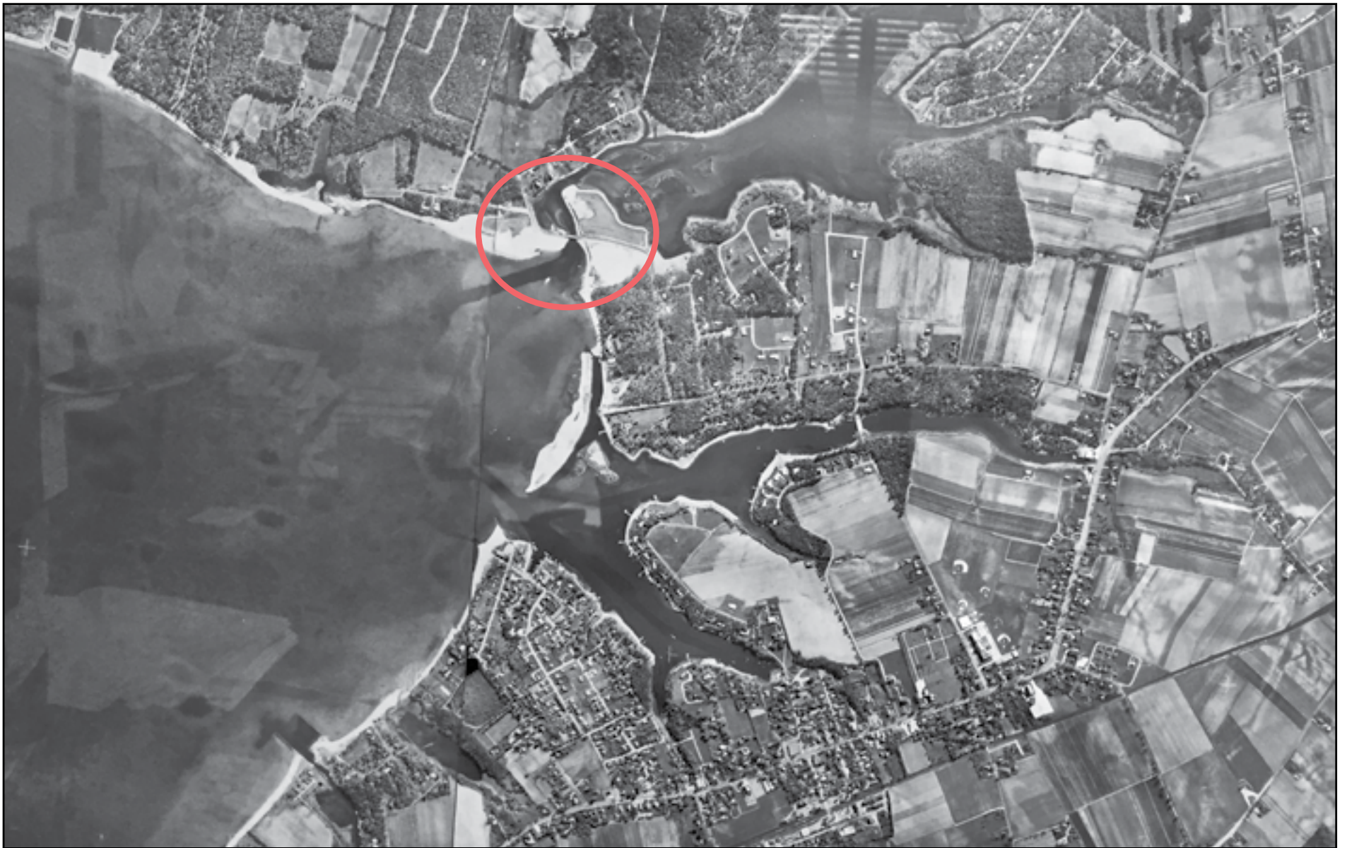
The circled area in this 1959 aerial view shows the terra firma on both sides of the north Bayview Road as seen in this issue.
