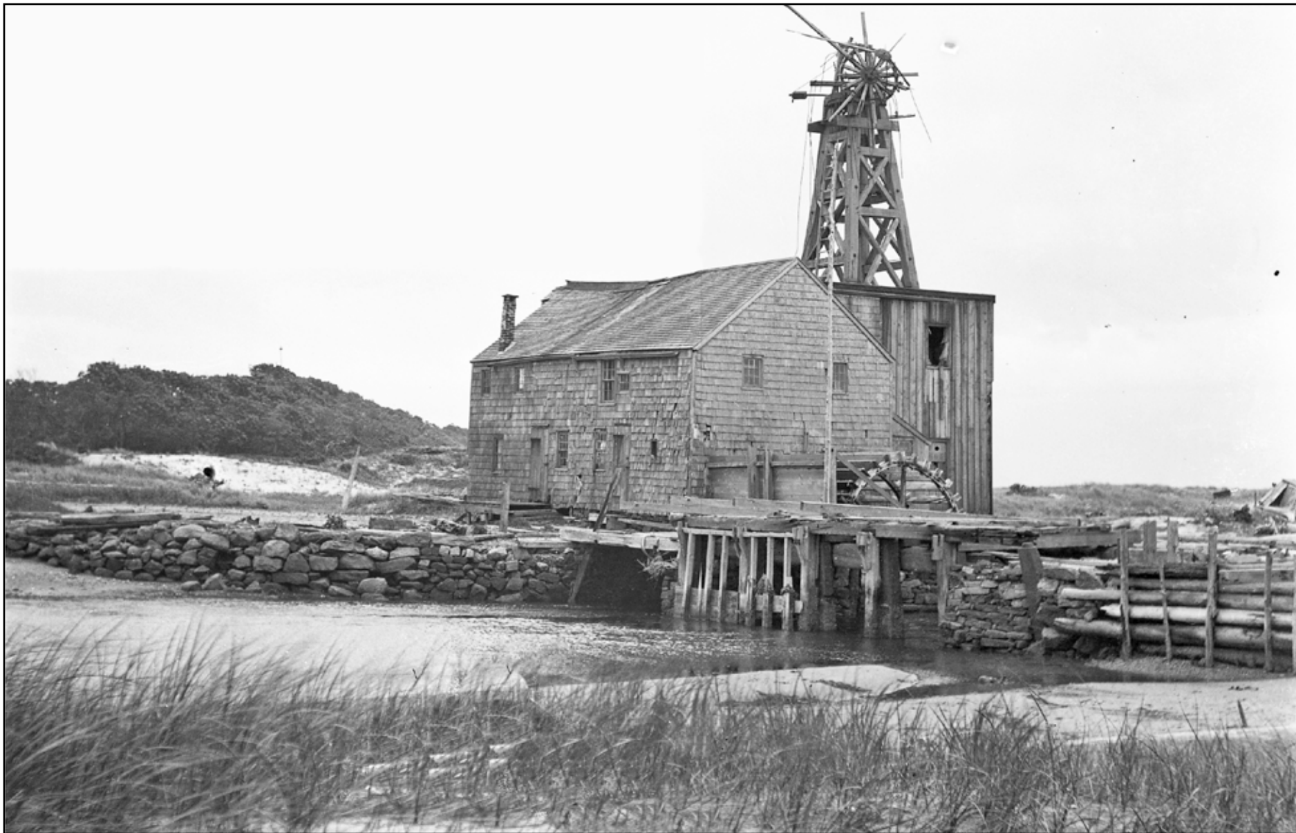
View of the Peconic Mill looking West.
