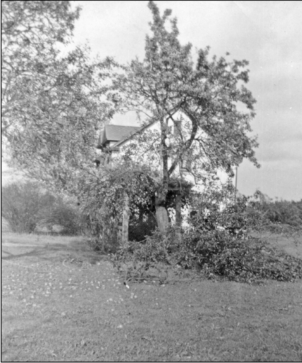
Garage and apartment structure on east side of property. Tree damage in front is a result of Hurricane Carol in 1954.
