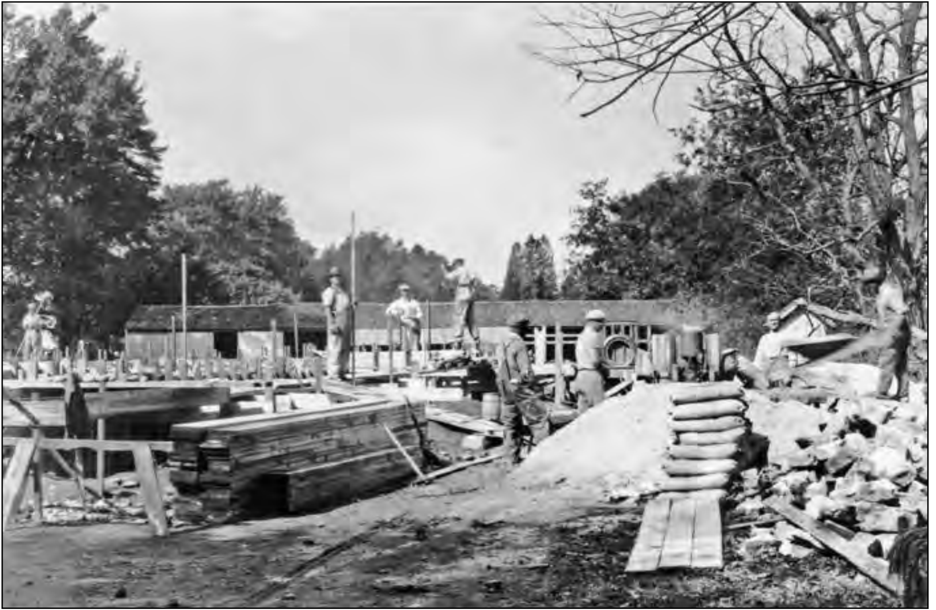
The rebuilding begins, as the forms are laid.
