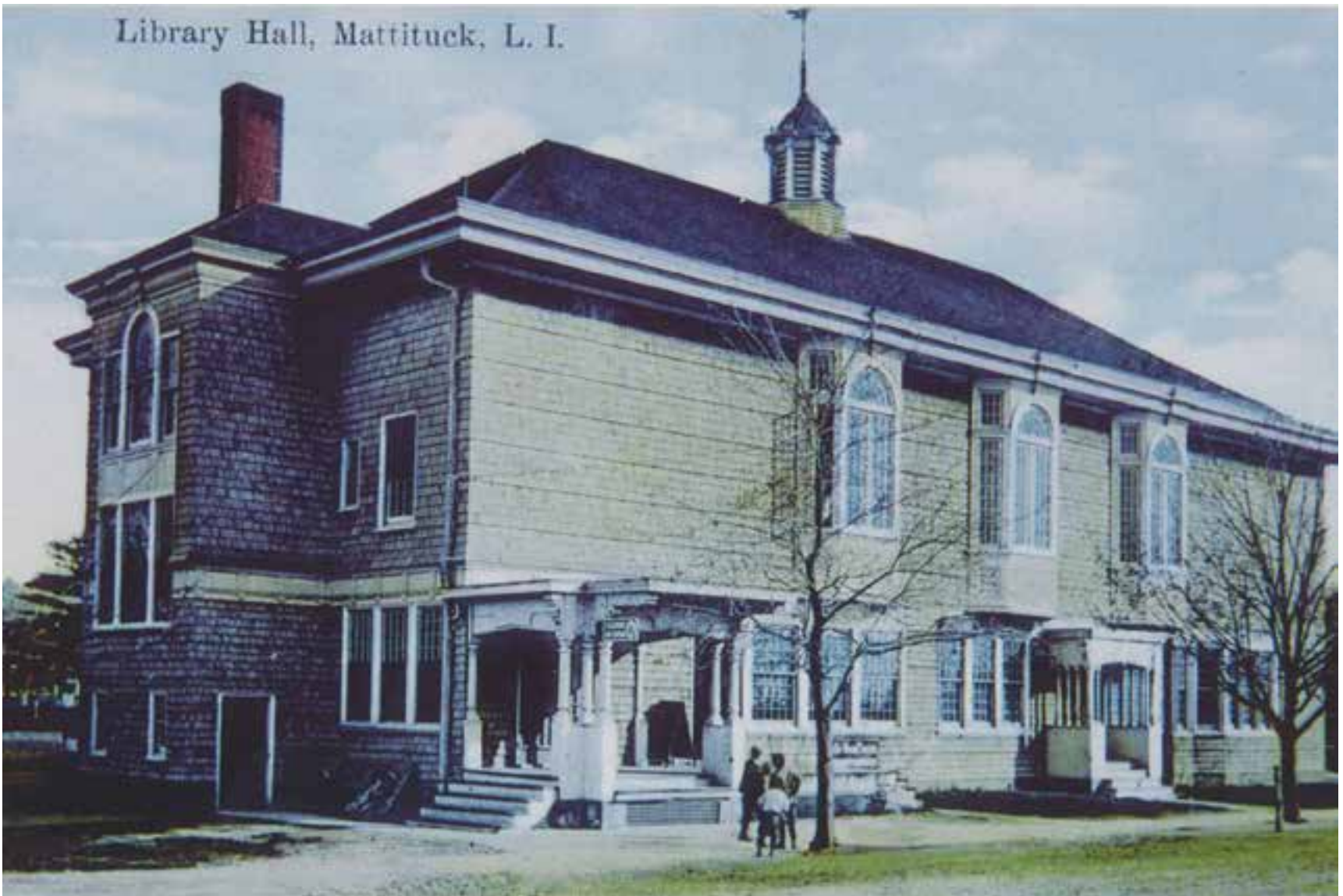
In 1916 extensive repairs were made in the Presbyterian Church, making it necessary to close it for three months while services were held in Library Hall, once located on the southeast corner of Pike Street and Westphalia Avenue, but torn down in 1963.
